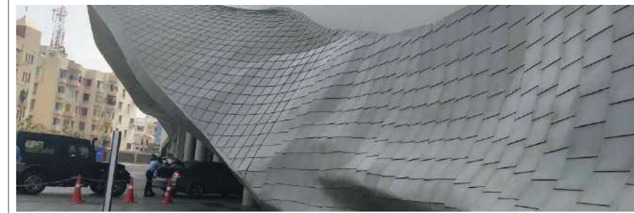
Project: Esplanade Mall, Bhubaneswar Aspect: QUARTZ Strat System: VMZ Parametric Panel
